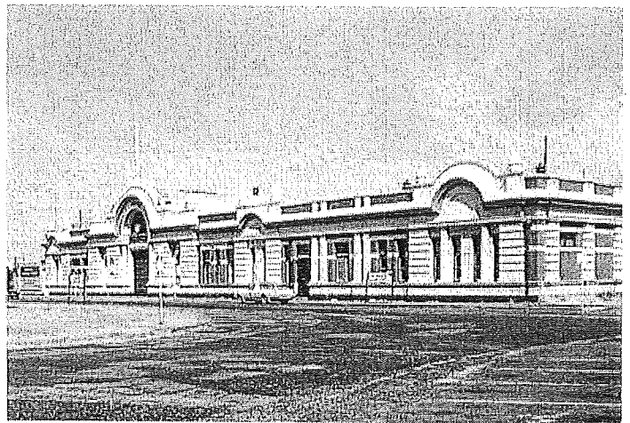
Fremantle Railway Station, 01.01.1979 (Courtesy HCWA web site)
