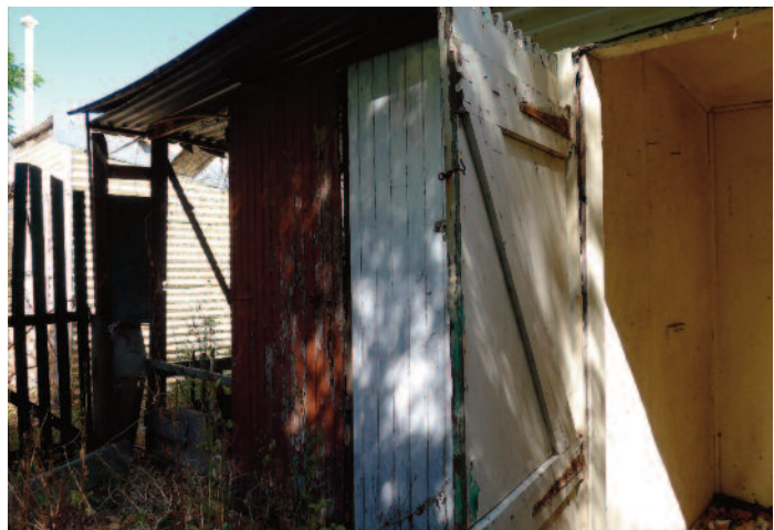
Rear sheds of warders' cottages
