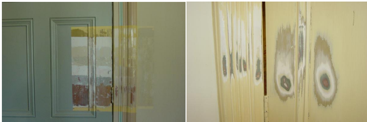
Paint ladders & scrapes reveal previous colour schemes National Trust of Australia (WA) Head Office - The Old Observatory, West Perth
