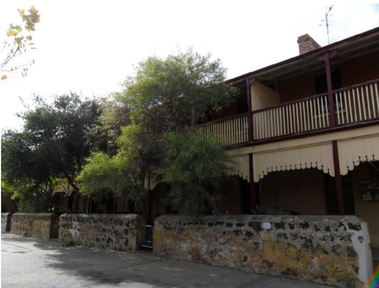
Photo 3: View across Henderson Street Mall of W3 partially obscured by plantings in the small front yards behind the low front limestone wall.
