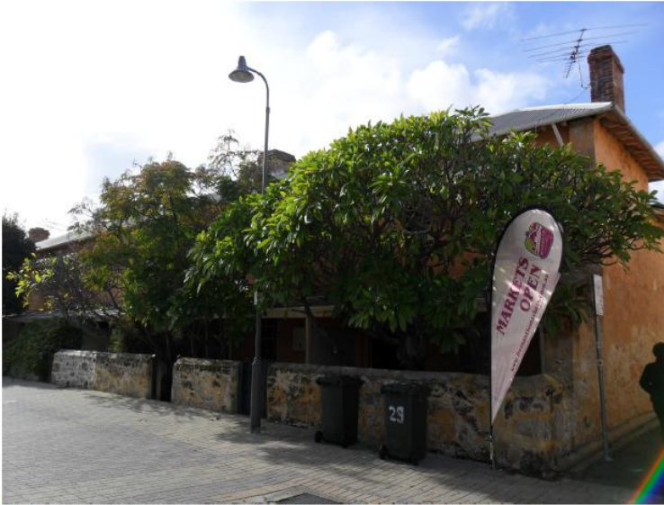
Photo 5: View across Henderson Street Mall of the front and south side of W1 adjacent to the laneway entrance to the Fremantle Markets.
